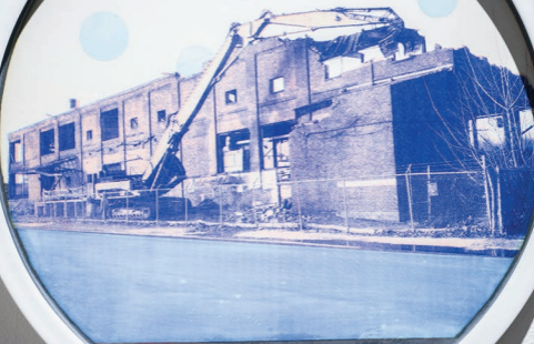
GE Building 2 underway Lima City
